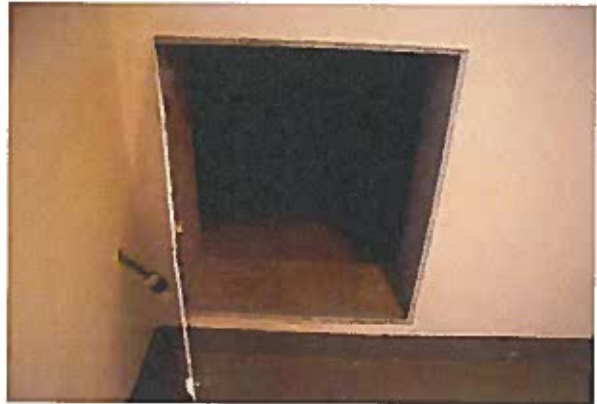
Photo 34 - Access to Ceiling/Ductwork Coating
