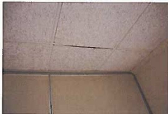
Photo 12 - Drop Ceiling Tile
