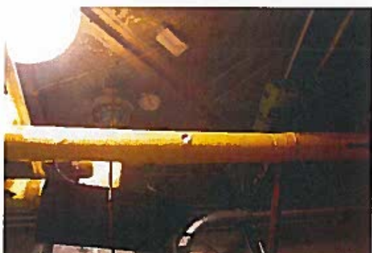
Photo 8 - Pipe Wrap Yellow
