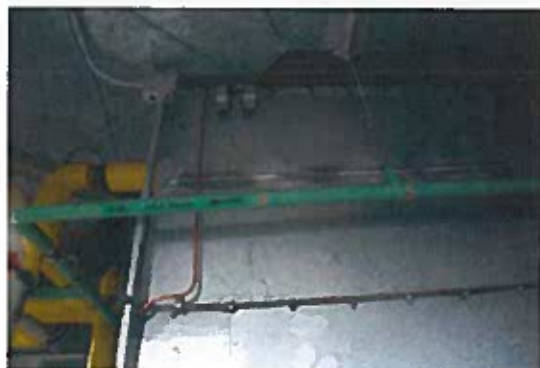
Photo 7 - Pipe Wrap Green
