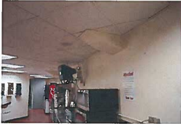
Photo 33 - Drop Ceiling Tile
