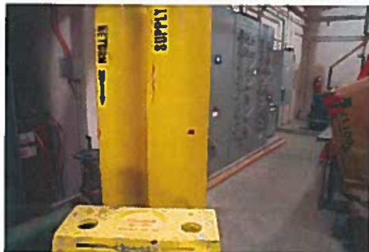
Photo 20 - Pipe Wrap Yellow
