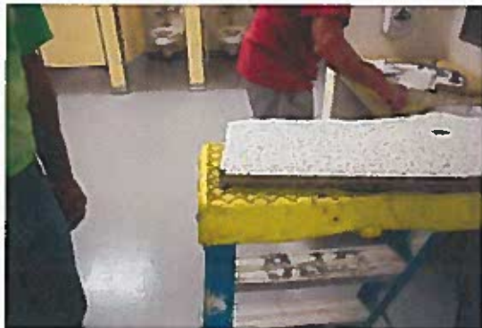
Photo 3 - Drop Ceiling Tile
