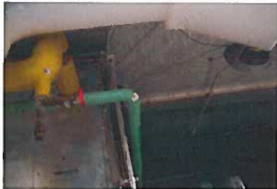
Photo 5 - Elbow Insulation Green
