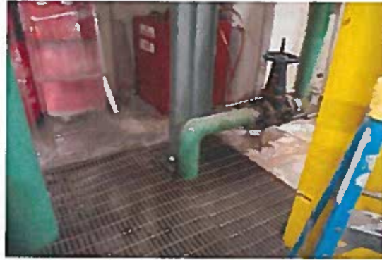
Photo 18 - Elbow Insulation Green
