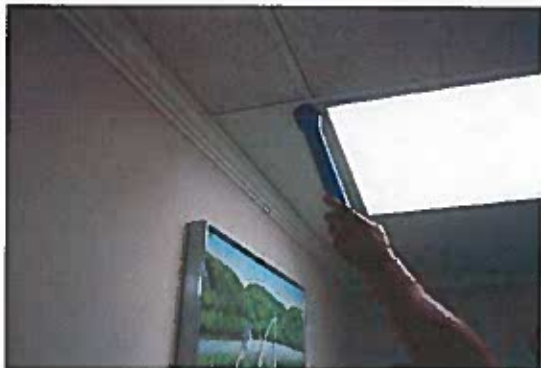
Photo 14 - Drop Ceiling Tile
