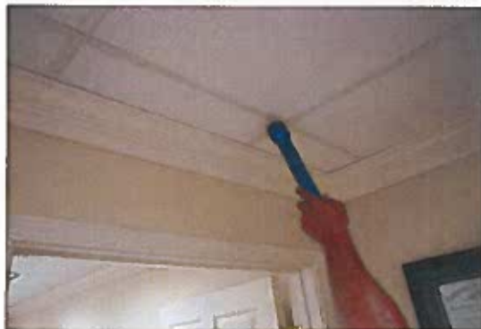
Photo 13 - Drop Ceiling Tile
