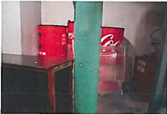
Photo 19 - Pipe Wrap Green
