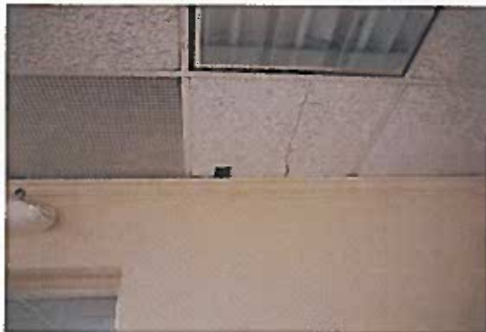
Photo 11 - Drop Ceiling Tile
