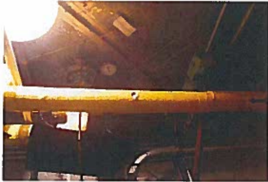
Photo 9 - Pipe Wrap Yellow
