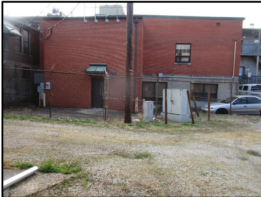
Subject Building Rear View
