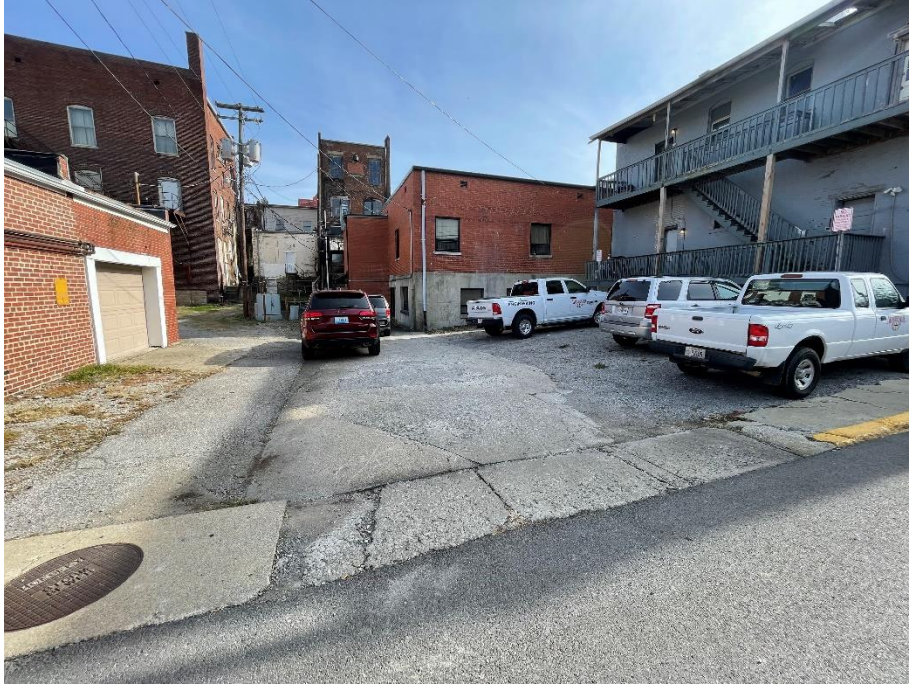
EXTERIOR VIEW AND DRIVE OF SUBJECT PROPERTY
