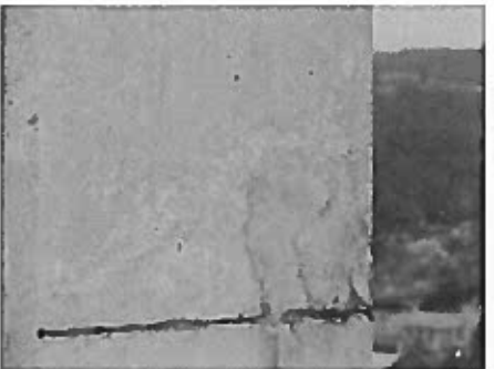
Existing Concrete Patches
