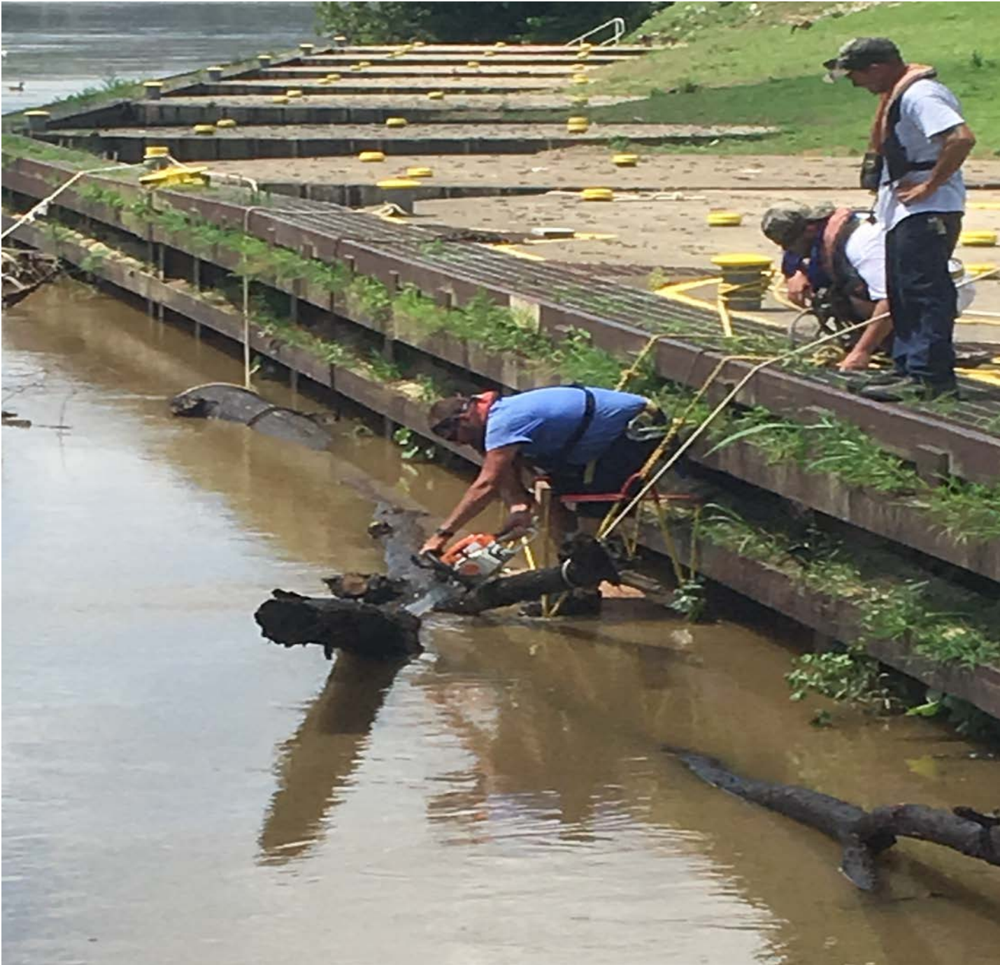
Lock and Dam 4, Lockmasters removing drift after high water
