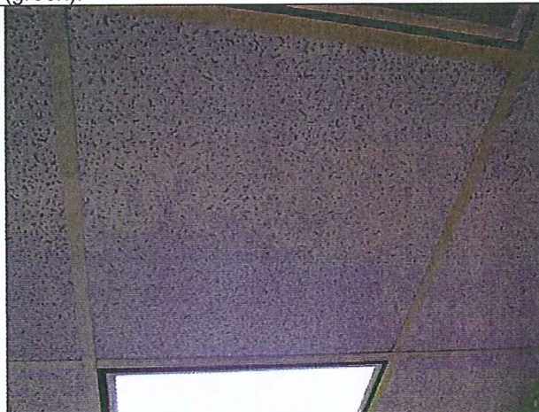
Photograph #17: Sample CT-Lobby-2: 2'x2' Drop Ceiling Tile.
