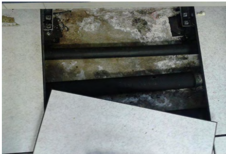
Photo 3 Black foam insulation Fourteenth Floor
