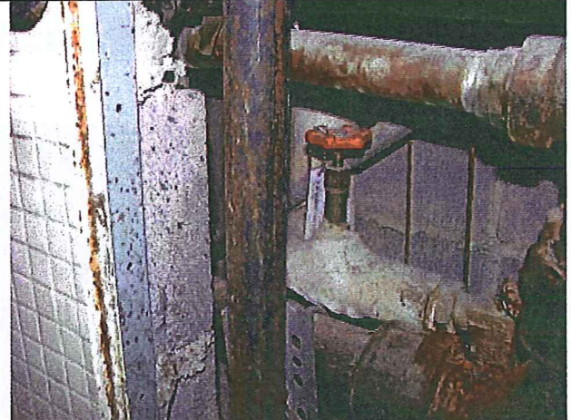
Photograph #10: Sample CT-5: 3" Pipe Joint Compound.
