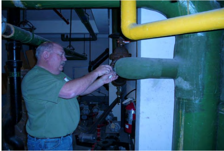
Sample 31 Pipe wrap Floor 13A
