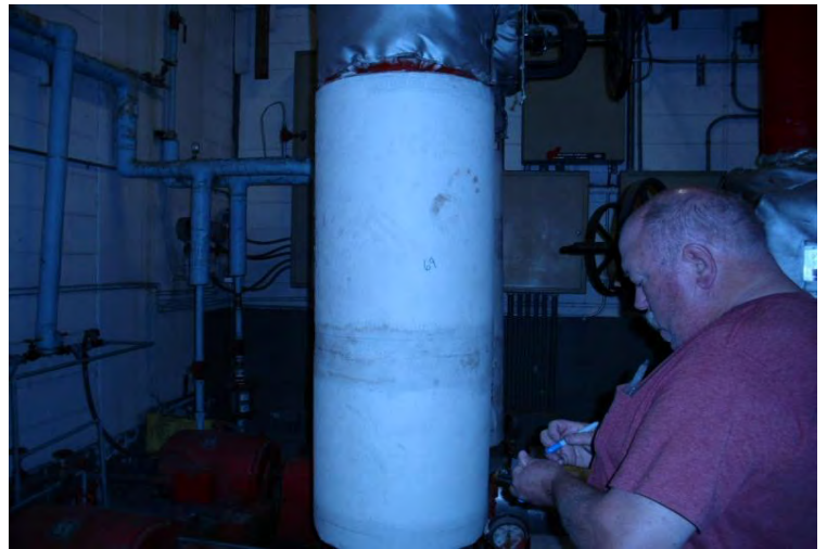
Sample 69 Pipe wrap Boiler Room
