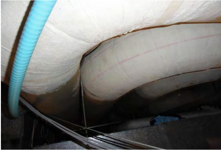
Sample 135 Pipe wrapping Crawl Space
