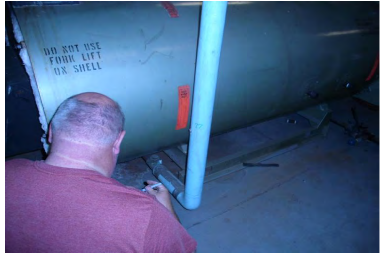
Sample 77 Pipe wrap Boiler Room
