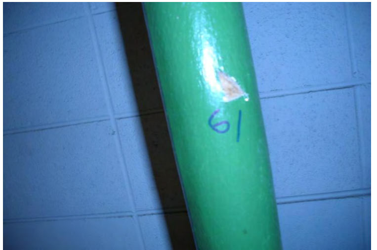
Sample 61 Pipe wrap Ground floor
