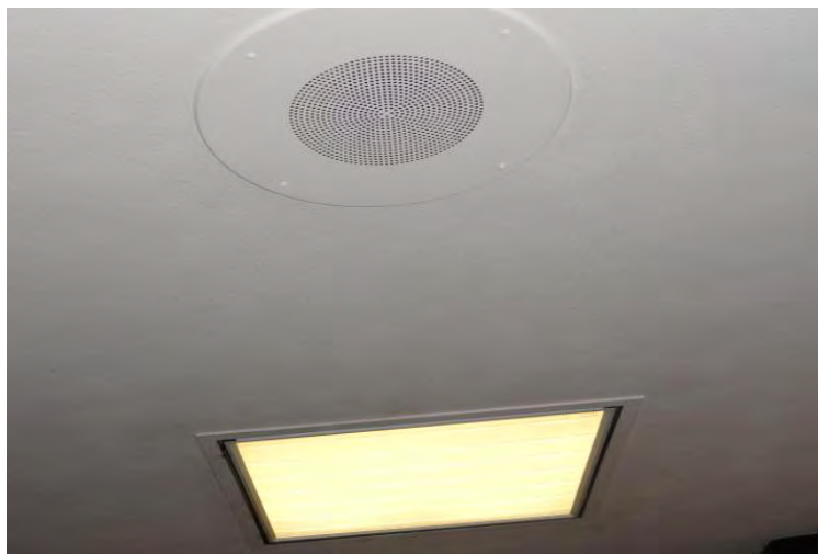
Sample 118 Ceiling tile Floor 17
