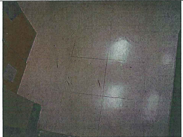
Photograph #16: Sample CT-Lobby-1: 12" Floor Tile (white).
