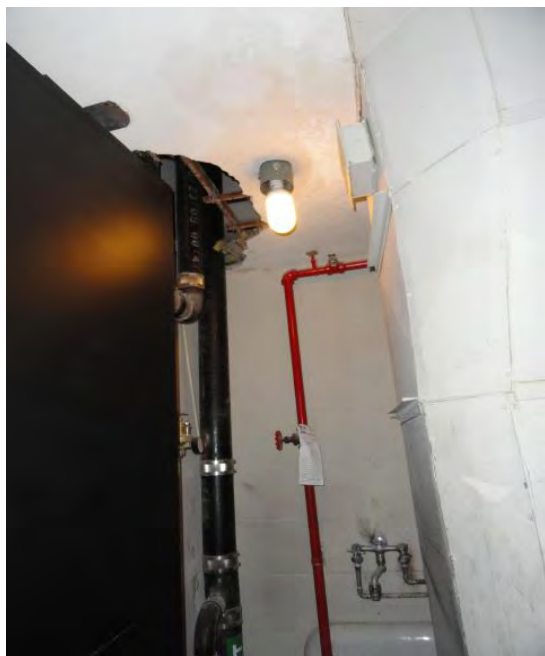
Sample 111 Ceiling tile Floor 21
