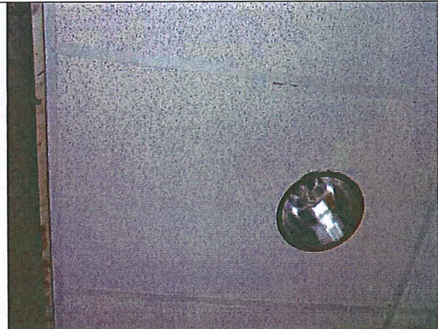
Photograph #18: Sample CT-Mez-1, CT-Mez-2 & CT-Mez-3: 2'x4' Drop Ceiling Tile.
