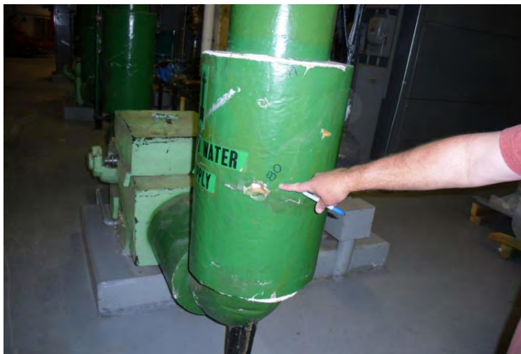
Sample 80 Pipe insulation Mechanical Room
