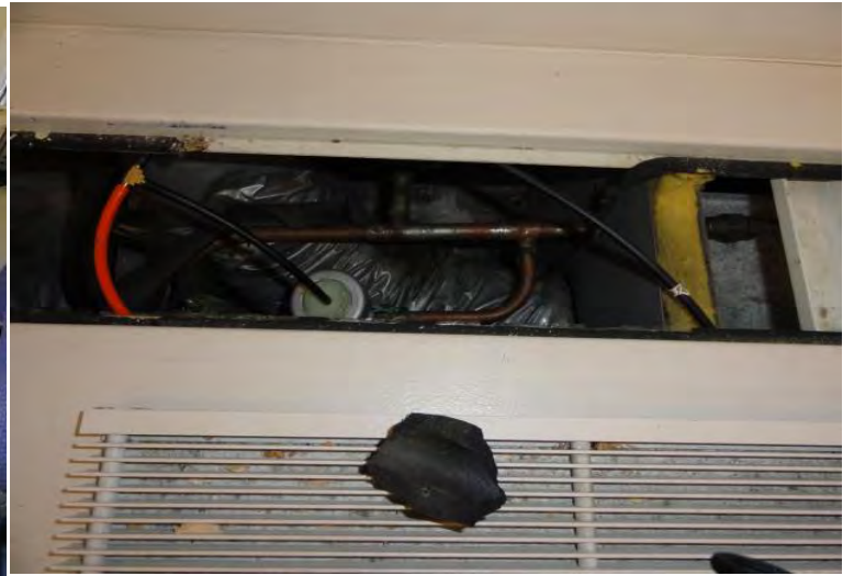
Sample 101 Water unit insulation Floor 1
