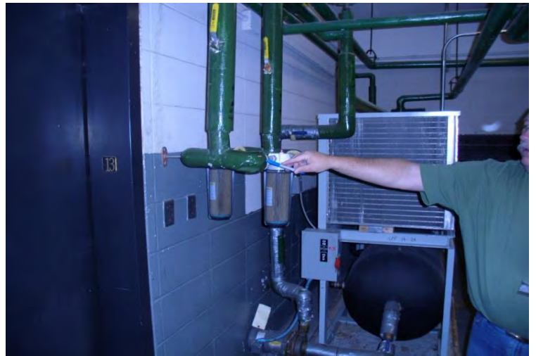
Sample 34 Joint Floor 13A
