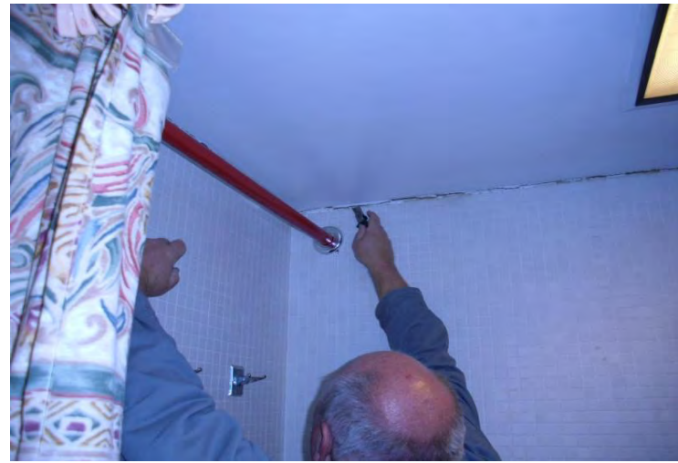
Sample 97 Ceiling covering Ground floor
