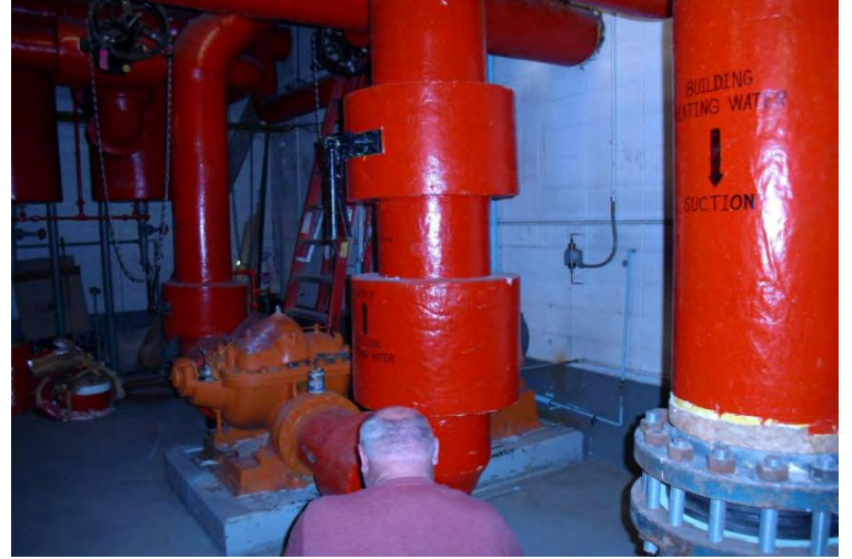
Sample 83 Pipe insulation Mechanical Room
