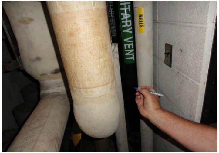
Sample 51 Pipe Wrap Floor 13B
