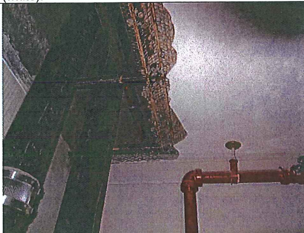
Photograph #3: Sample CT-23-1: Plaster Ceiling
