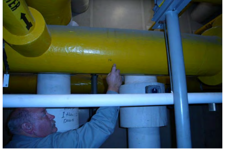
Sample 16 Pipe wrap Floor 13A
