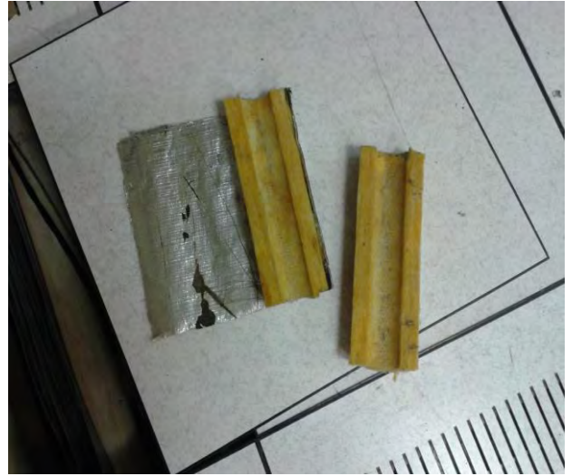
Photo 2 Insulation foil and pipe insulation Fourteenth Floor
