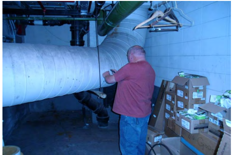
Sample 63 Vent tape Ground floor
