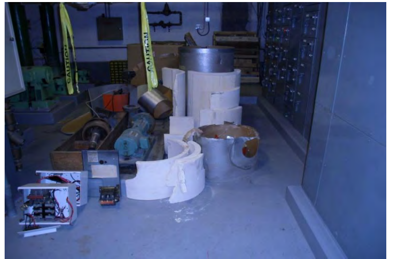
Sample 85 Loose thermal Mechanical Room
