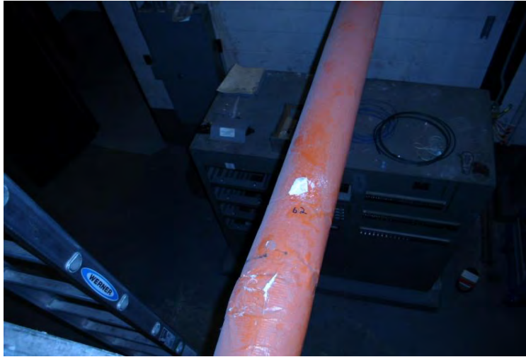
Sample 62 Pipe wrap Ground floor
