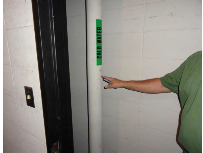
Sample 49 Pipe Wrap Floor 13B
