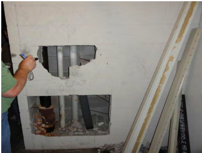
Sample 50 Pipe Wrap Floor 13B
