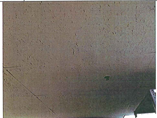
Photograph #22: Sample CT-Mez-14, CT-Mez-15 & CT-Mez-16: 2'x4' Drop Ceiling Tile.
