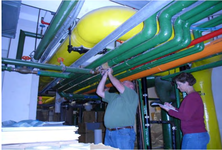
Sample 39 Pipe insulation Floor 13A
