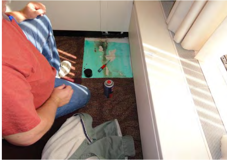
Sample 105 Floor tile covered with carpet Floor 5
