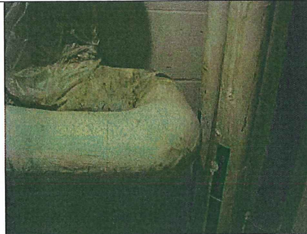
Photograph #11: Sample CT-6: 6" Pipe Joint Compound.
