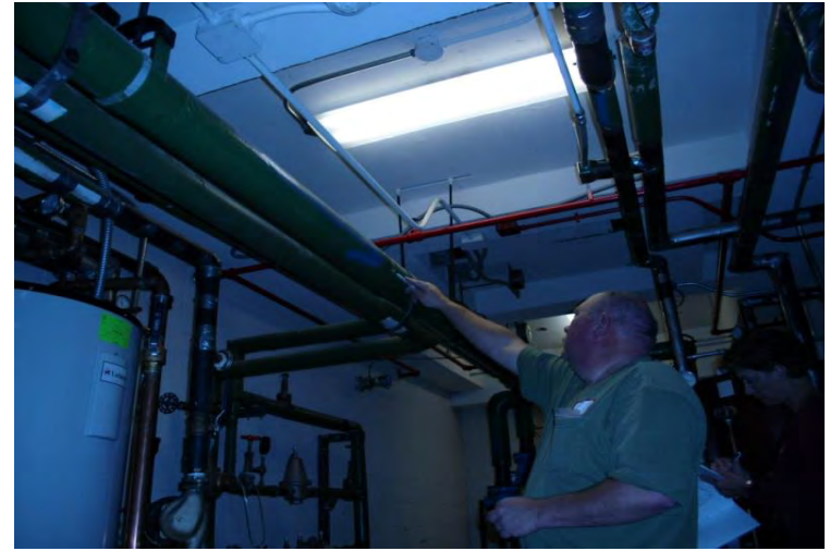
Sample 42 Pipe wrap Floor 13A
