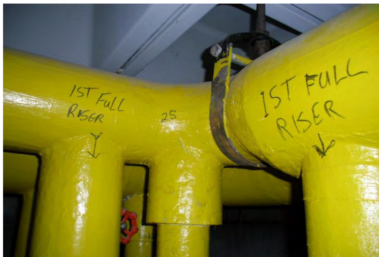
Sample 25 Joint Floor 13A
