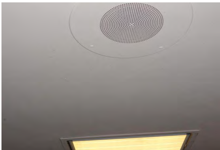
Sample 129 Ceiling texture Floor 9
