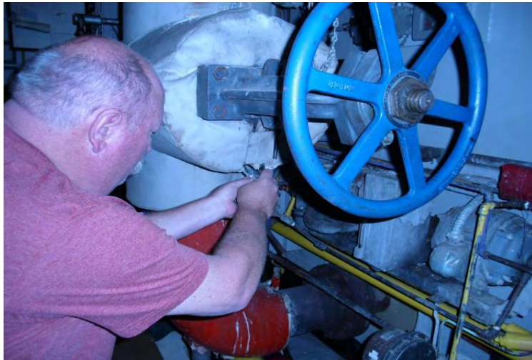
Sample 78 Over pack Boiler Room
