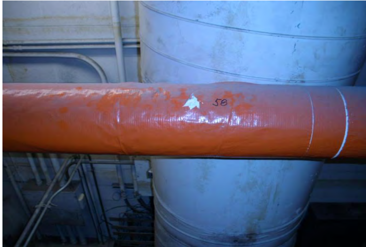
Sample 58 Pipe wrap Ground floor
