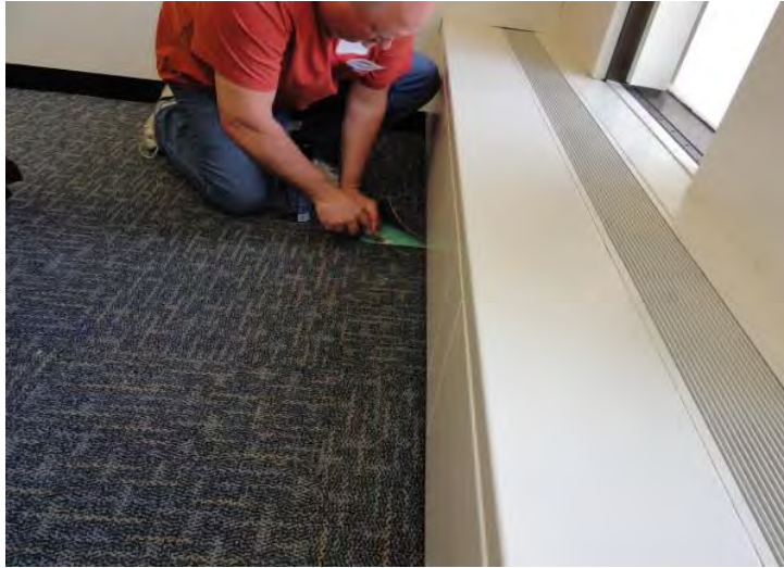
Sample 104 Floor tile covered with carpet Floor 4
