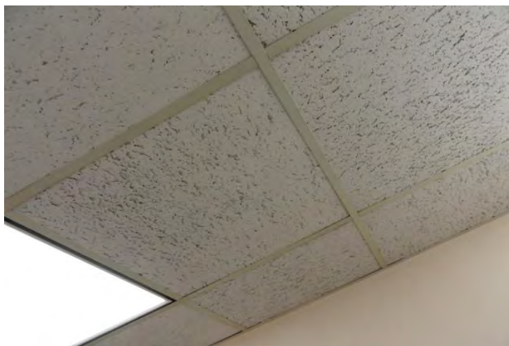
Sample 122 Ceiling tile Floor 15
