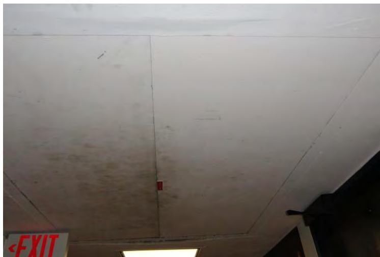
Sample 106 Ceiling plaster Floor 24
