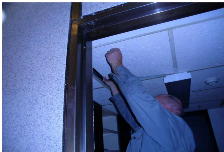
Sample 92 Ceiling tile Ground floor
