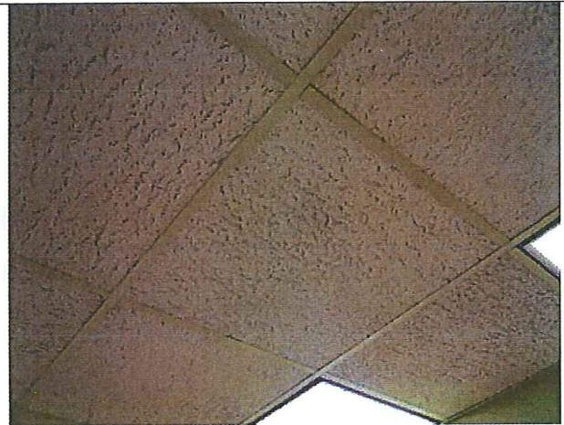
Photograph #2: Samples CT-24-2, CT-24-3 & CT-24-4: 2'x2' Drop Ceiling Tile
