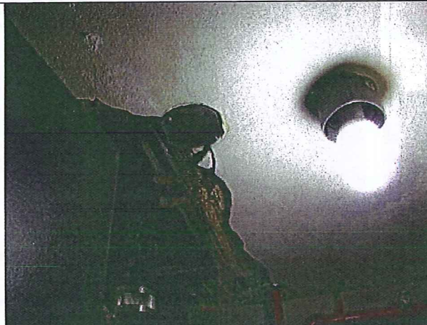
Photograph #9: Sample CT-4 & CT-9: Plaster Ceilings.
