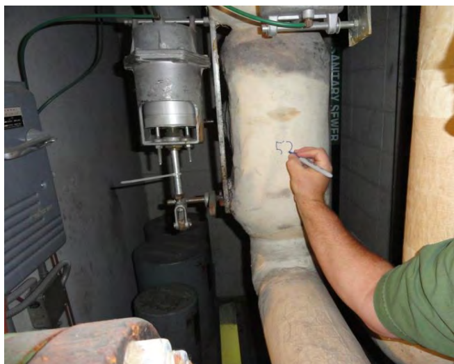
Sample 52 Pipe Wrap Floor 13B
