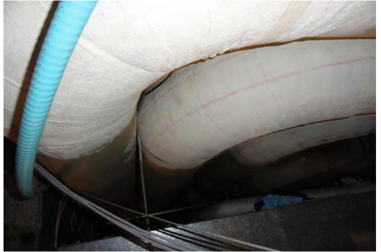
Sample 136 Piping insulation Crawl Space
