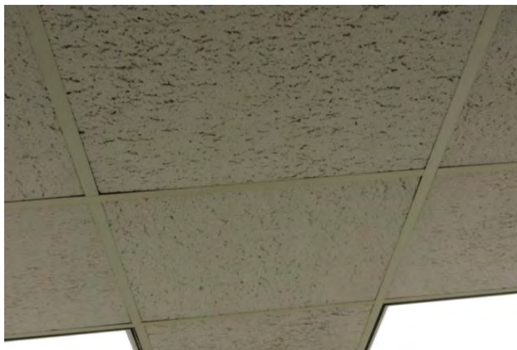
Sample 116 Ceiling tile Floor 18
