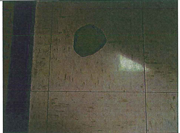
Photograph #20: Sample CT-Mez-7, CT-Mez-11, CT-Mez-12 & CT-Mez-13: 12" Floor Tile (white with brown streaks)
