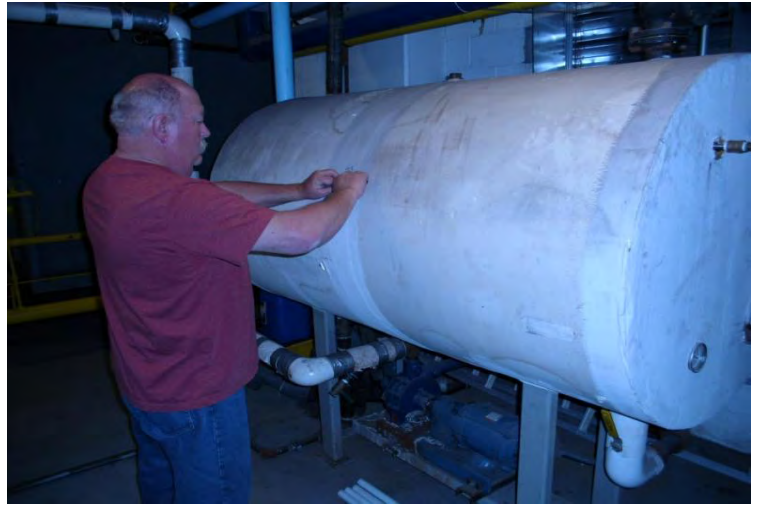
Sample 73 Tank insulation Boiler Room
