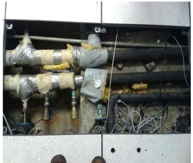
Photo 4 Joint compound Fourteenth Floor
