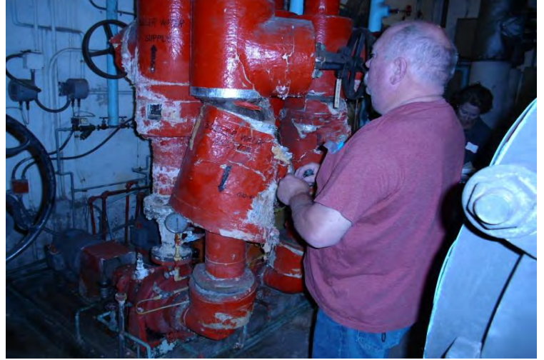
Sample 71 Pipe wrap Boiler Room
