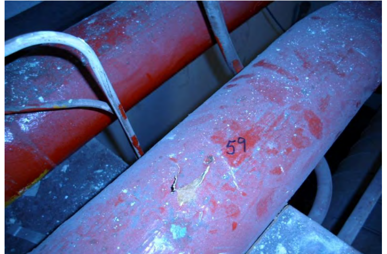
Sample 59 Pipe wrap Ground floor
