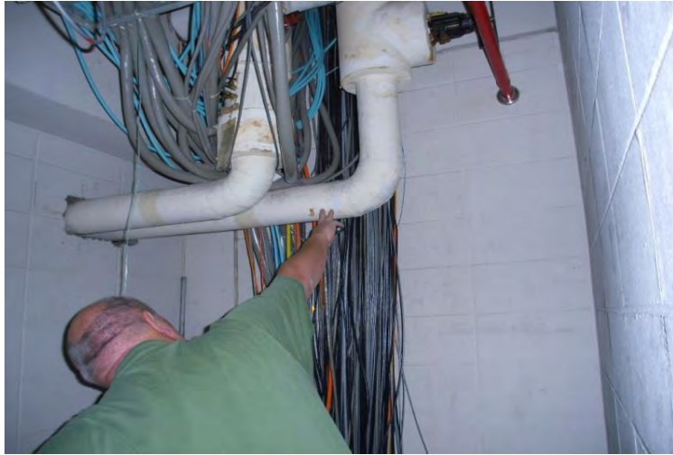
Sample 48 Pipe wrap Floor 13B
