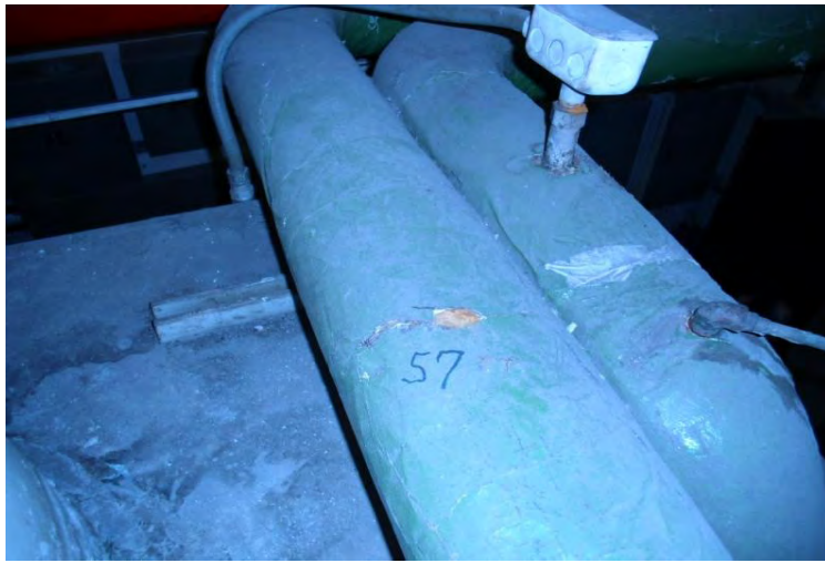
Sample 57 Pipe wrap Ground floor
