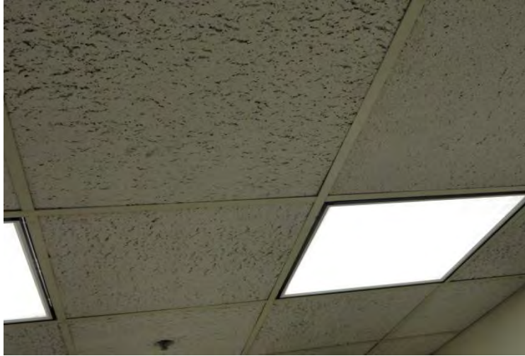
Sample 115 Ceiling tile Floor 19
