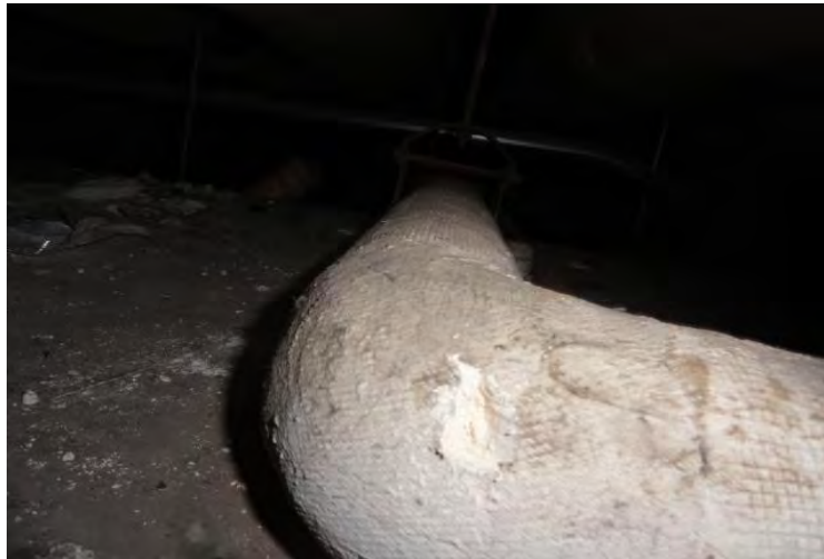
Sample 137 Elbow Crawl Space
