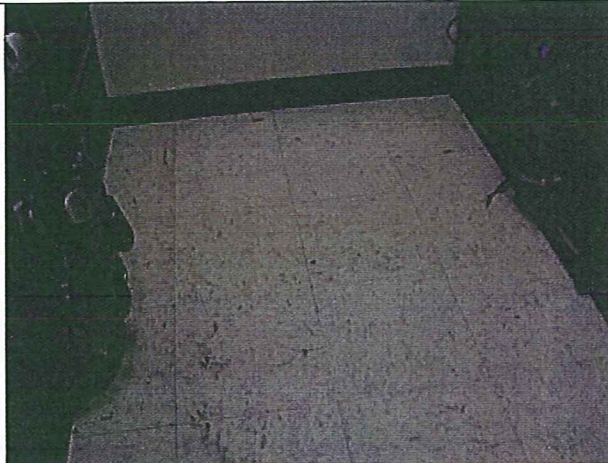
Photograph #7: Sample CT-2 & CT-7: 12" white floor tile with black mastic.
