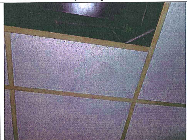
Photograph #24: Sample CT-Ground-4, CT-Ground-5 & CT-Ground-6: 2'x2' Drop Ceiling Tile.
