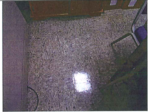
Photograph #4: Sample CT-15-1, CT-15-2 & CT-15-3: 12" Floor Tile (grey).
