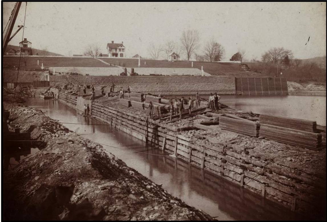
Repairs to timbercrib dam at Lock No. 3 circa 1901. Courtesy of the National Archives.
