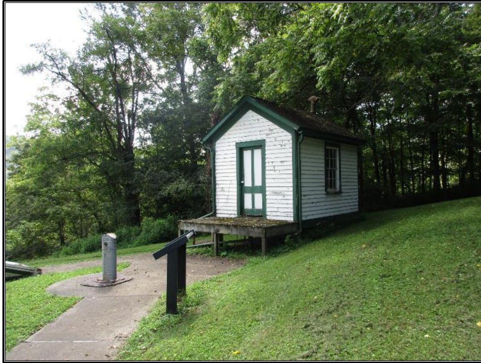
Image 12. View of the upper lockhouse laundry house, circa 2016. Courtesy of Cultural Resource Analysts, Inc.
