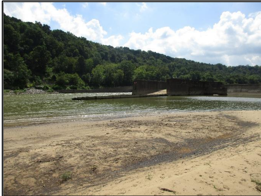
Image 4. View of Lock and Dam No. 10 from downriver, circa 2016. Courtesy of Cultural Resource Analysts, Inc.
