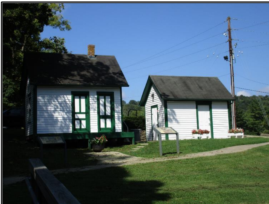
Image 11. View of the lower lockhouse laundry building and coal house, circa 2016. Courtesy of Cultural Resource Analysts, Inc.
